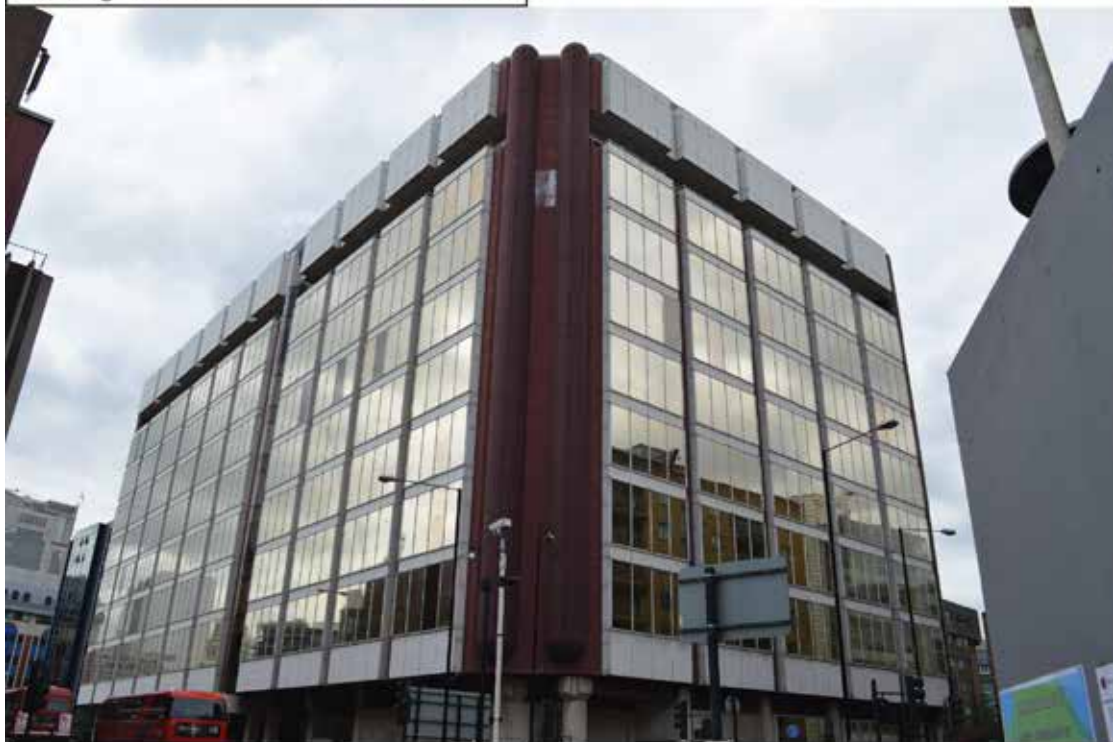
CASE No. 16/00209/FULMAJ Looking northwest from Goodman's Yard
