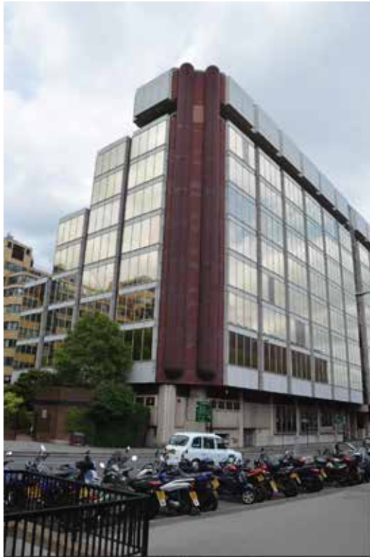
CASE No. 16/00209/FULMAJ Looking northeast from Goodman's Yard
