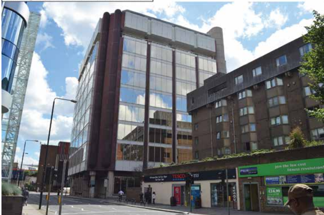
CASE No. 16/00209/FULMAJ Looking southwest from Mansell Street
